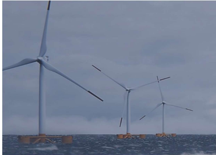
Digital rendering of Dolfines floating offshore wind platform with turbines in situ. Image courtesy of Dolfines.
